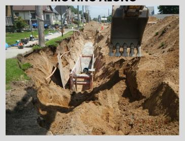
Work continues on this year's major infrastructure project: the \$3.5 million reconstruction of Roosevelt Avenue, including all underground utilities. Most of the new pipes—water, sanitary sewer, storm sewer—are now in the ground. Grading and graveling in preparation for the concrete paving should start in August.
