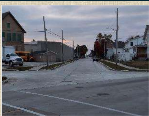
Narrowed up 12th Street and Roosevelt Street intersection, note that School Street now intersects just into Roosevelt Street not a huge 5-street intersection.
