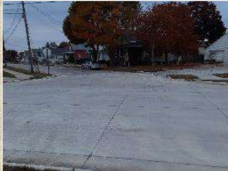
Narrowed up 9th Street and Roosevelt perpendicular intersection verses the original skewed intersection
